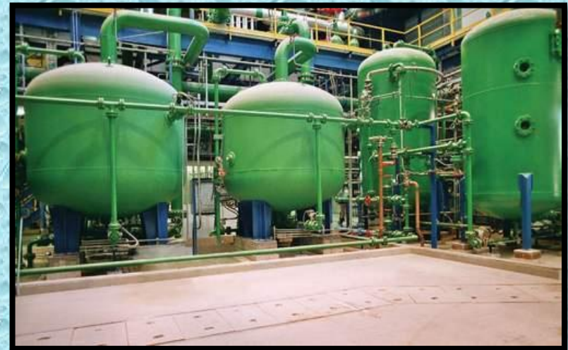
Condensate Polishing Unit
