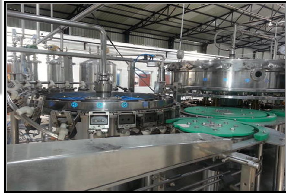
CARBONATED SOFT DRINK PLANT
